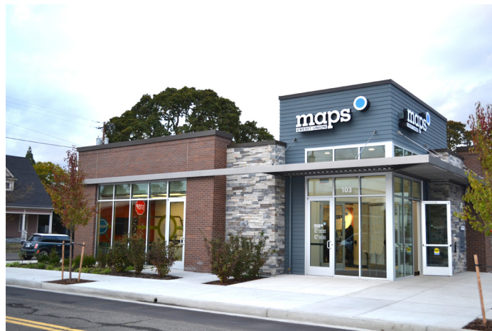
New Silverton Branch location
